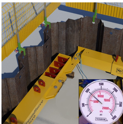
13. With all legs now connected, open the lock off valve and pressurise the brace against the trench sheets to approximately 1000psi (~70bar # ) unless otherwise stated.
