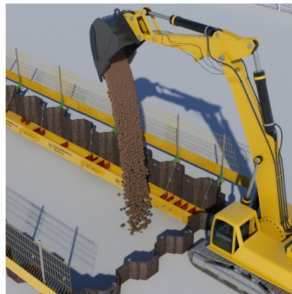
5. Continue backfilling and compacting to the underside of the top frame.
