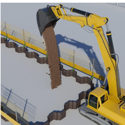
7. Reinstatement can then continue to ground level.
