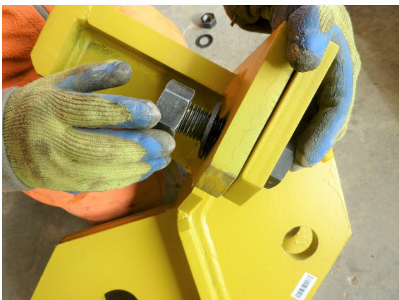
1. The Rough Adjuster Adaptor and Plinth is connected using 2 No. M30 nuts, bolts and washers.
