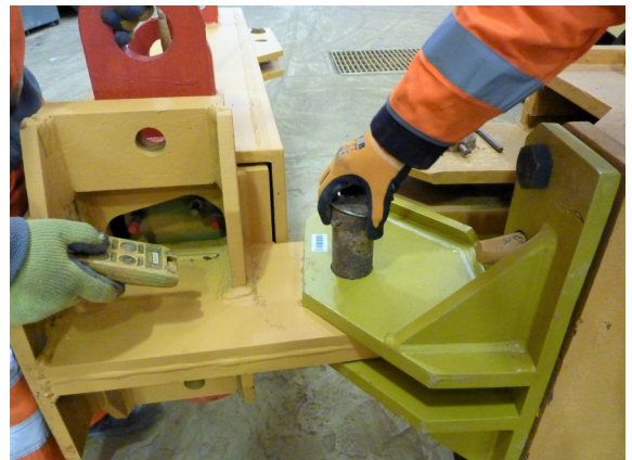
5. Secure using a Ref 6 - 60mm dia pin and R Clip. (see next page for complete connection)
